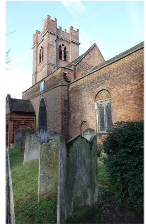
St. Luke's Church, Charlton Rebuilt 1630
